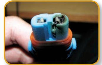
Melted Original-style Unit
